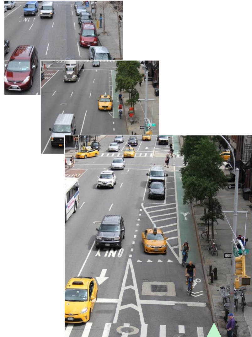
Progression of bicycle facilities on 2nd Avenue (none, buffered bike lane, PBL with Mixing Zone)
