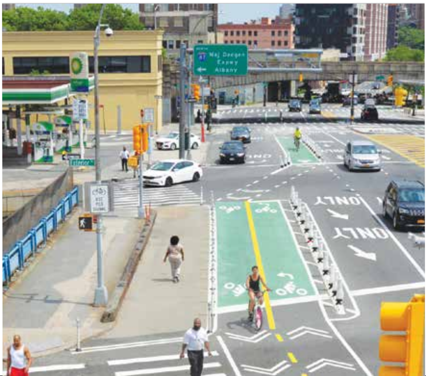
Protected Bicycle Connection with Painted Sidewalk Extension at 138th St in the Bronx
